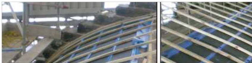
Roof insulation with va-Q-vip B
