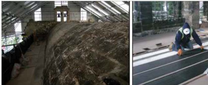
Roof insulation with va-Q-vip B
